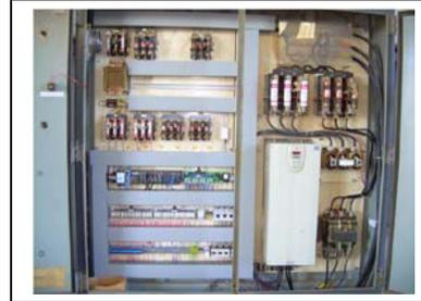
*Existing control cabinet and several existing components were incorporated into the new design to substantially reduce the project cost.*
